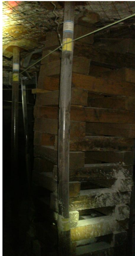
Figure 7.3: Steel support photogrammetry subject
