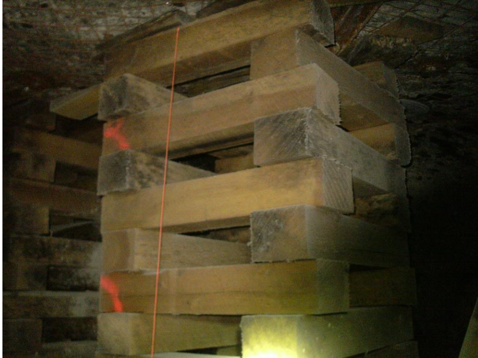
Figure 7.4: Wooden crib photogrammetry subject
