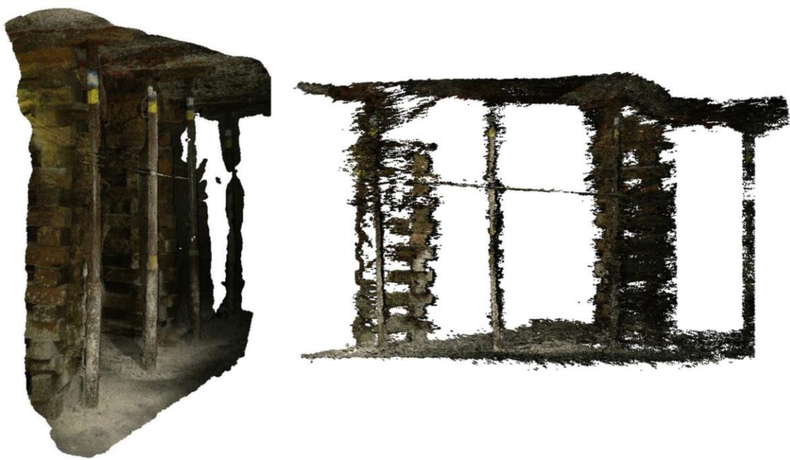
Figure 7.13: A reconstructed standing support triangulation from the camera position (left) and a dense point cloud as viewed perpendicular to the long axis of the crosscut (right).
