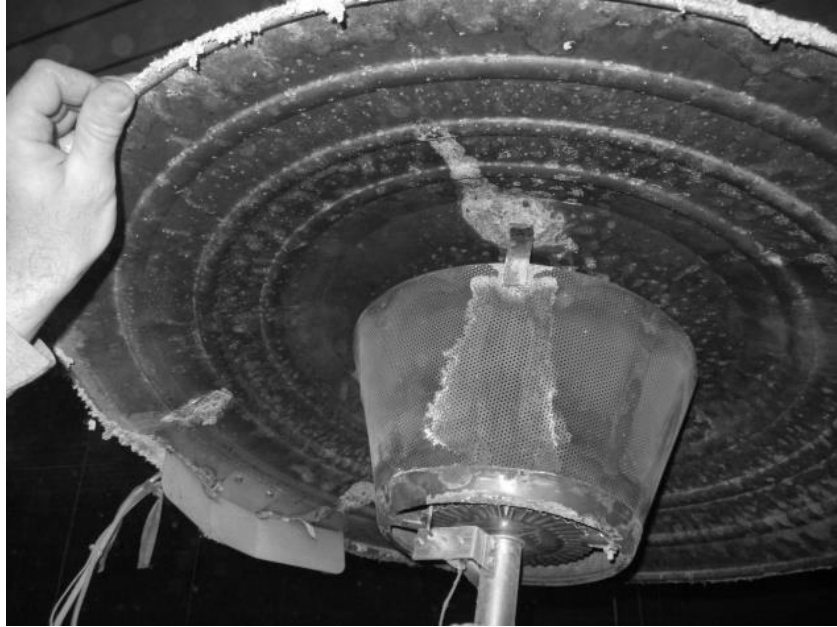
Figure 3.5. Damage to heater from PLT in reapplication house.
