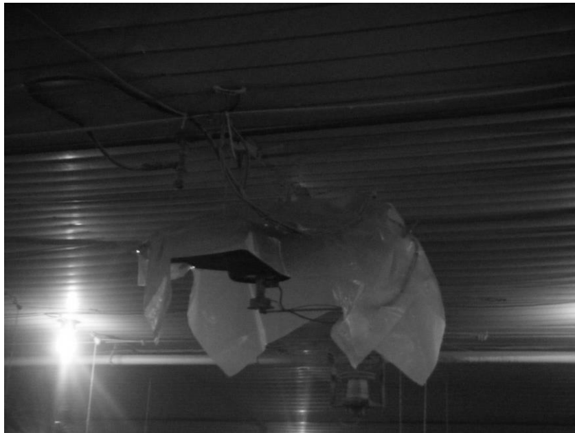
Figure 3.6. Plastic covering over heater in reapplication house.
