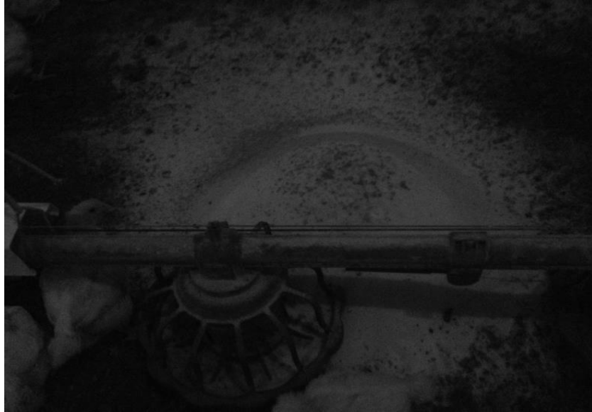
Figure 3.9. PLT deposit below spinner after fuse blowout in reapplication house.
