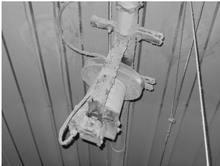
Figure 3.10. Spinner tilt causing distorted spread in reapplication house.
