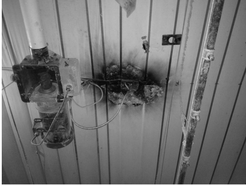
Figure 3.13. Melting of ceiling in reapplication house.
