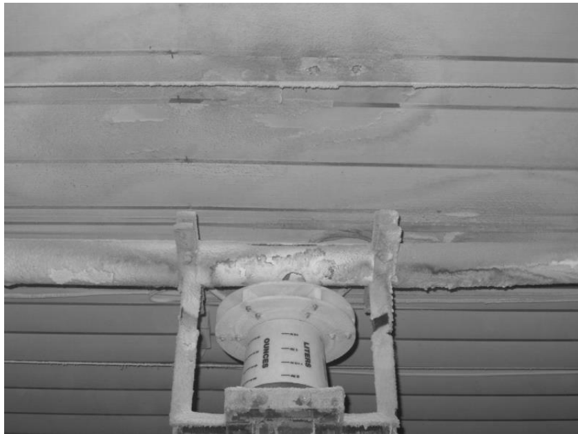
Figure 3.12. Holes in the ceiling above a spinner in reapplication house.
