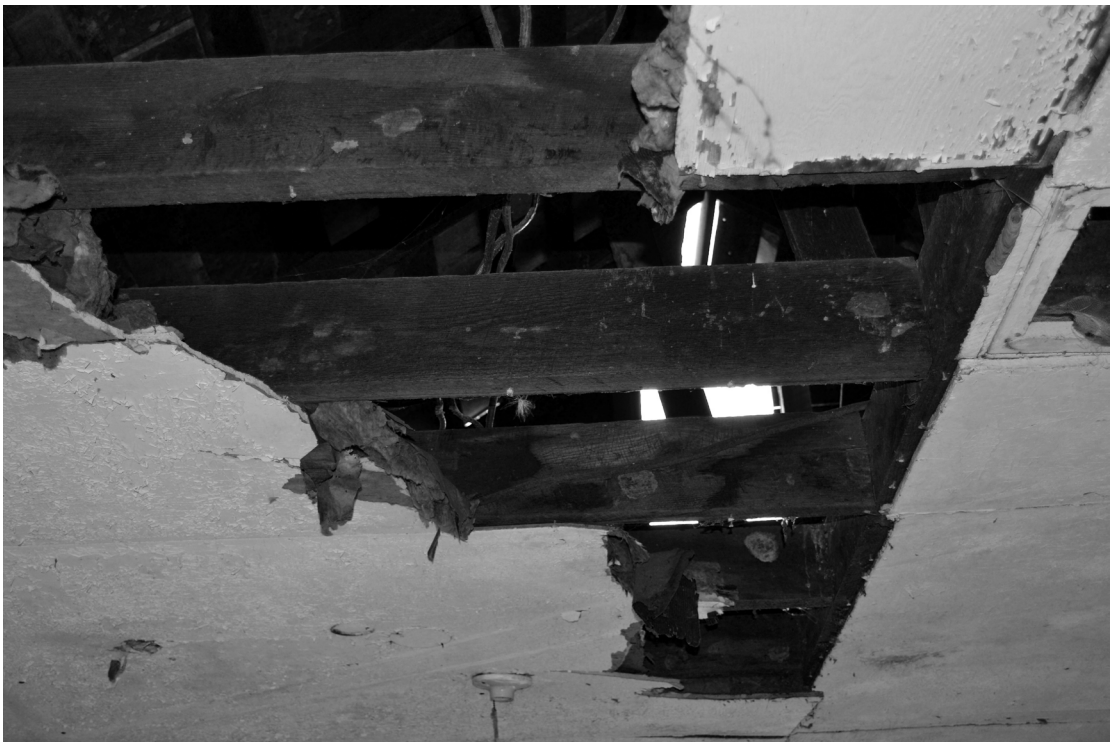
Details: Interior Roof
