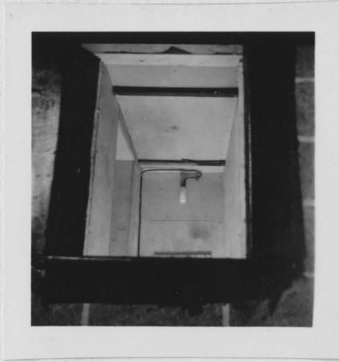
Figure 10 Interior of Freezer Compartment Note: Vapor Seal Around Opening.
