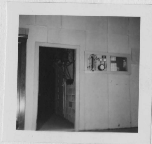
Figure 9 View of Control Board on Insulated Wall of Constant Temperature Compartment With Installed Unit in Background.
