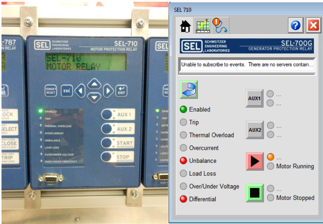
Figure 6.17 Motor Relay Home Screen
