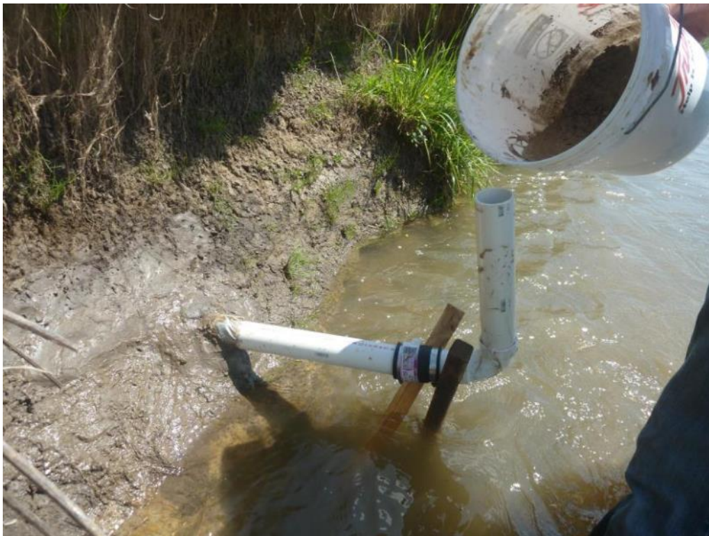
Figure D-4. The bank face is patched around apparatus and concrete is poured into the apparatus.
