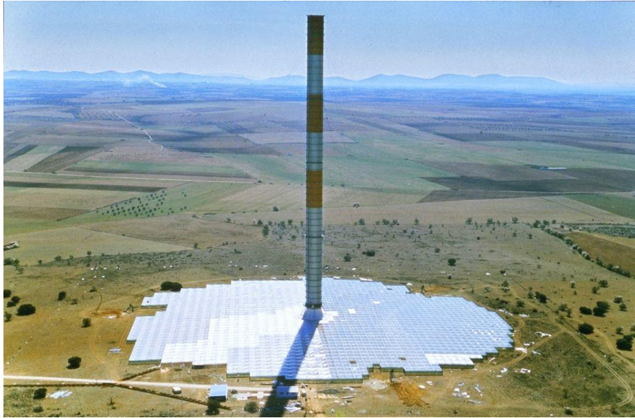
Figure 1.1 Prototype Solar Tower in Manzanares, Spain [3]
