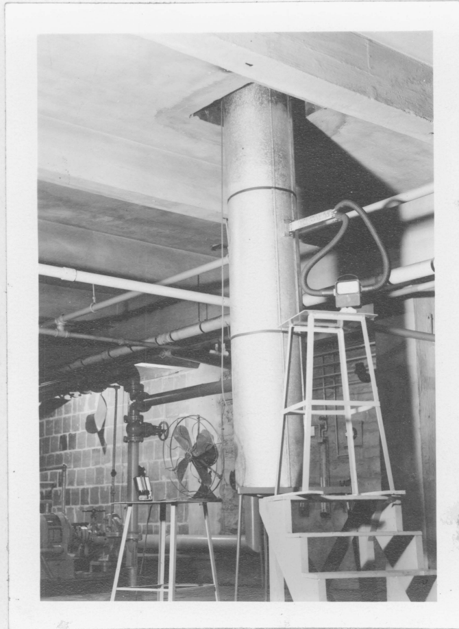
Fig. 5 - EIGHTEEN-INCH STACK WITH VELOMETER AND DUCT JET IN POSITION
