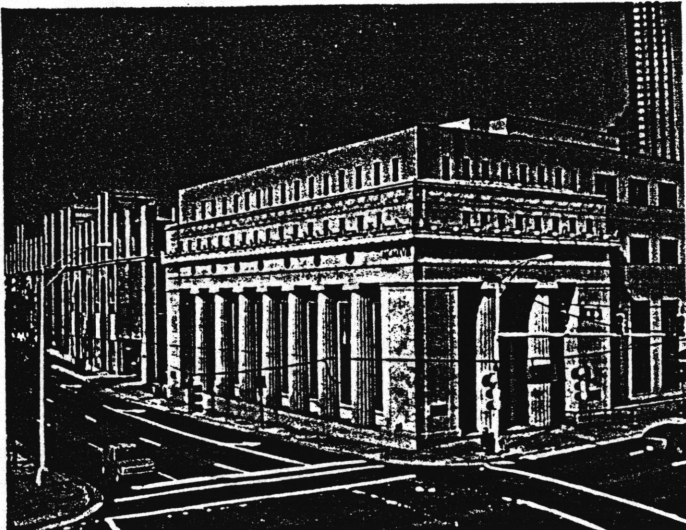
Charlotte National Bank parking deck 1988, Charlotte, N.C.
