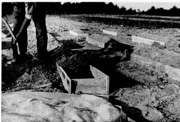
Figure 1. Field leaching frames at Chatham.
