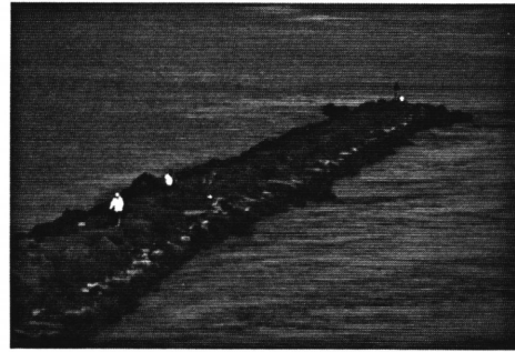
Stone groins, seaward bound; a slow deliberate construction of one block upon another
