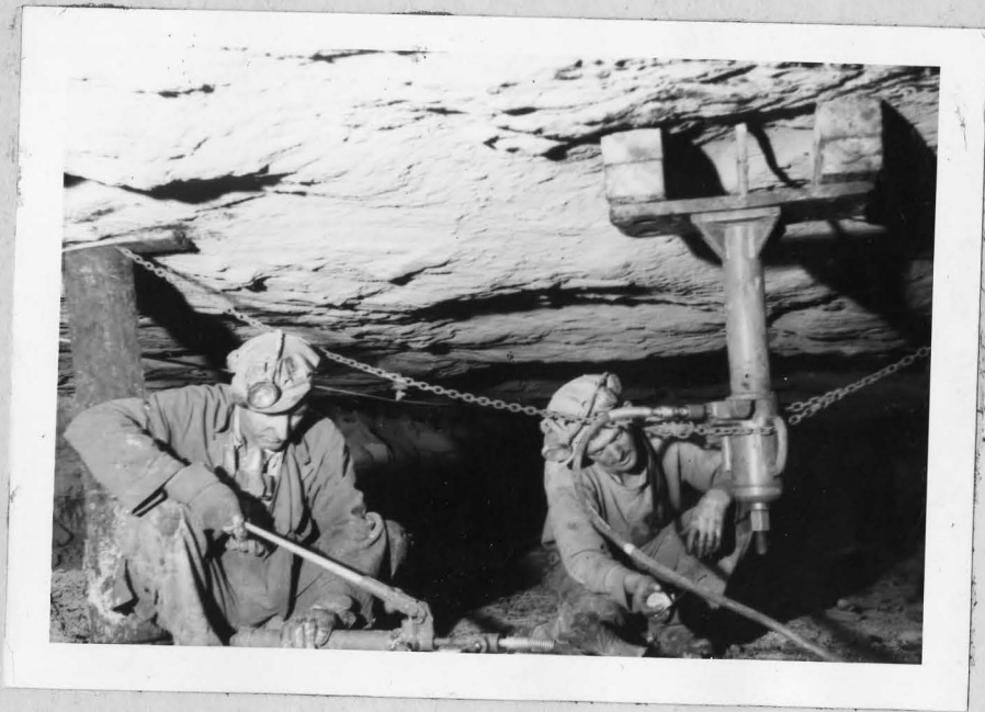
Figure 9. Installation of a Roof Bolt Pull Tester.
