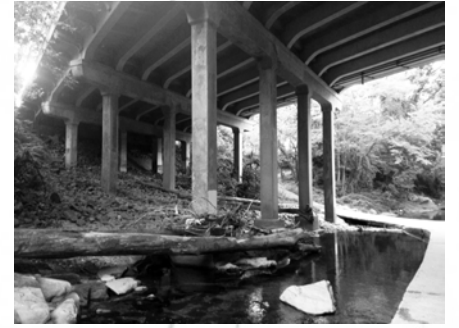
Bridge over the Site Four Mile Run & Columbia Pike
