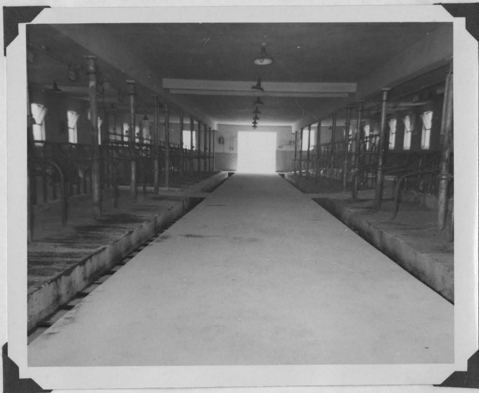
Figure 6. Photograph of Interior of Barn, showing mechanical gutter cleaner at lower left.
