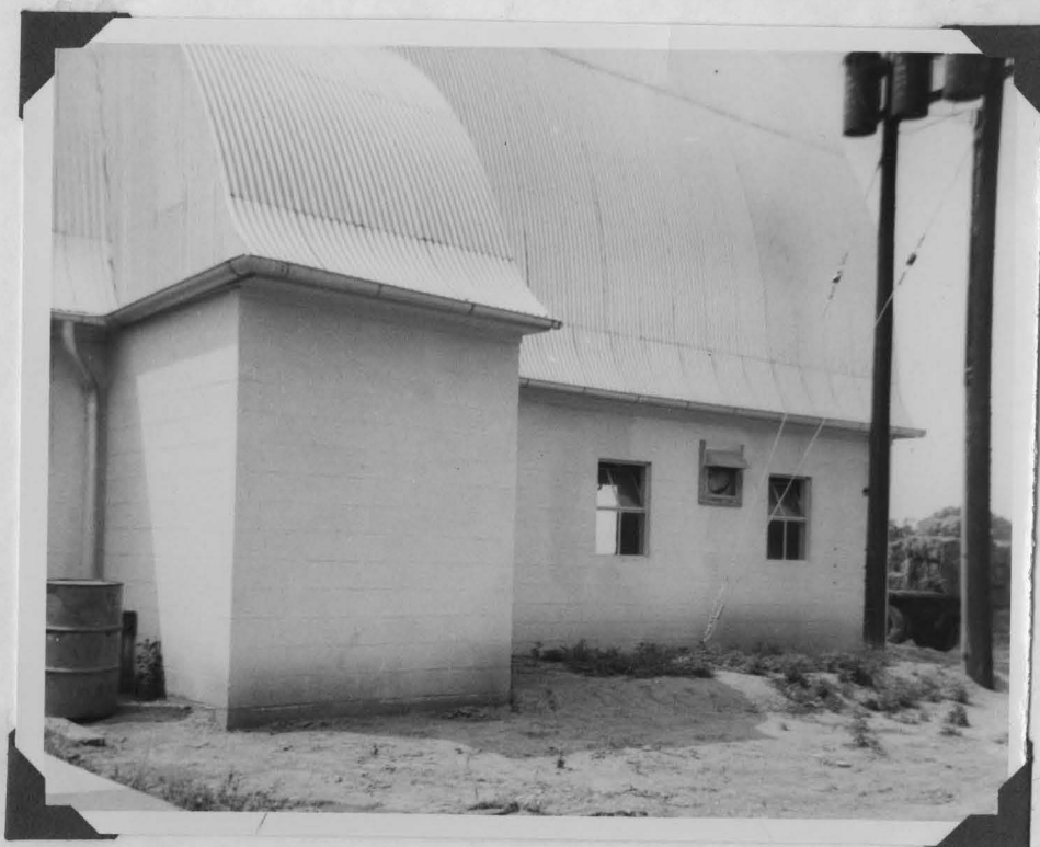
Figure 7. Photograph of Exterior of Barn showing hay chute attached to side of barn.
