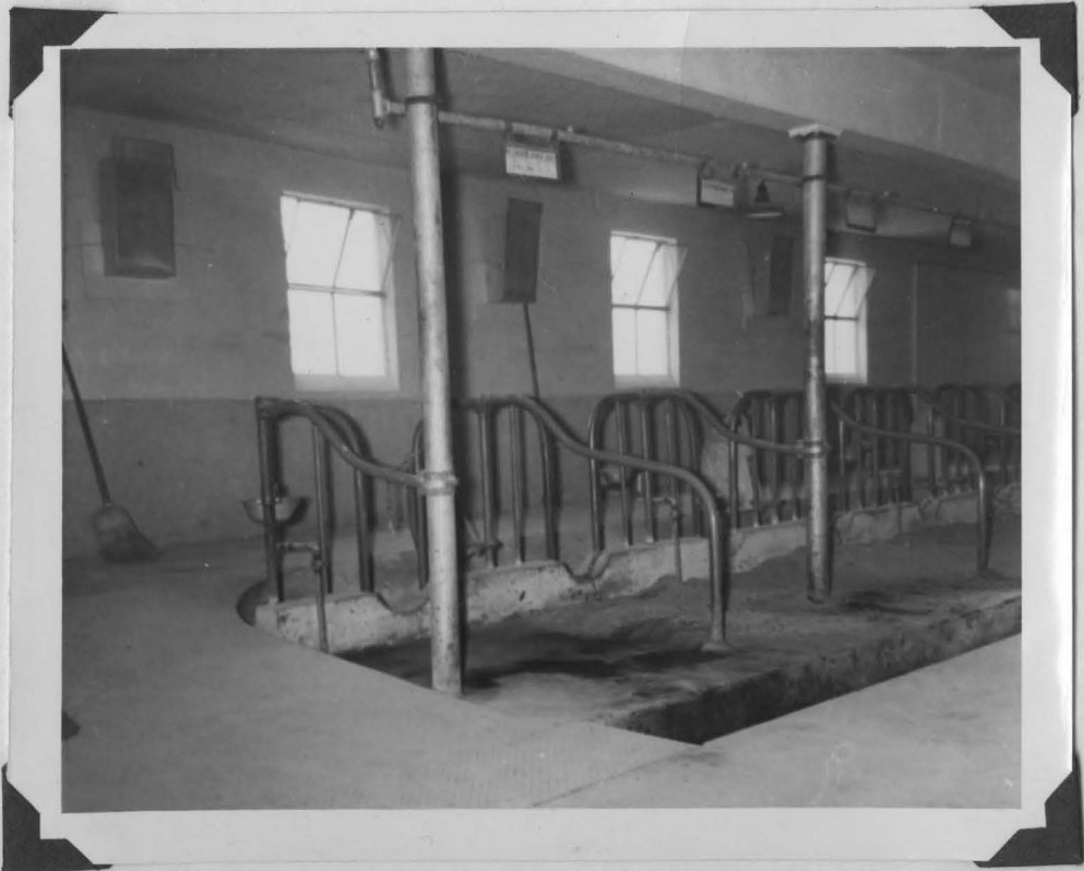
Figure 5. Photograph of Tie Stall.
