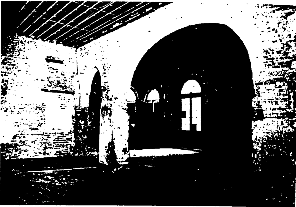
Figs. 139, 140. Cabildo: T) Original heavy timber roof trusses in third floor before the 1988 fire. (Courtesy Koch and Wilson Architects) B) Wide arch in corps de garde before 1966 archaeology work revealed a foundation pier. Original design of five arches restored by Wilson (Wilson and Huber 1973:106).
