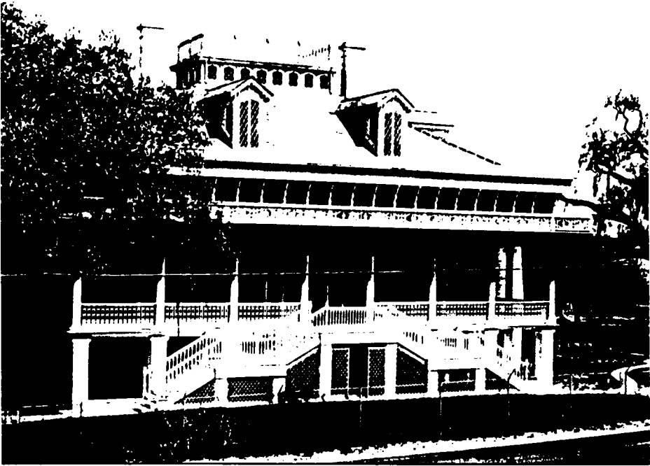
Figs. 149,150. T) San Francisco plantation house (ca. 1850) before restoration. Photograph by Abbye A. Gorin ca. 1960. B) After restoration (1973) by Koch and Wilson Architects. (Courtesy Koch and Wilson Architects)
