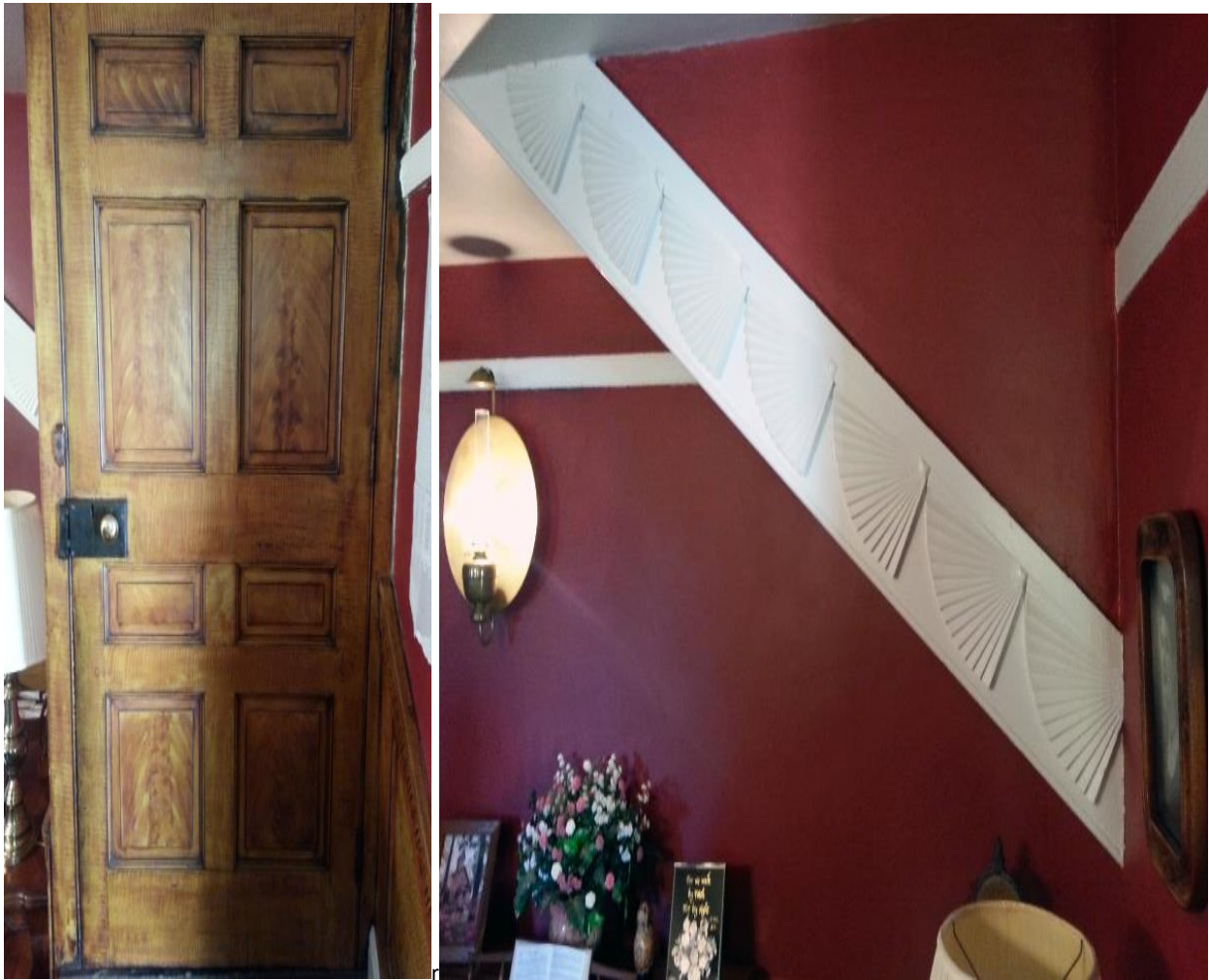
Figure 65: Entrance to Half-Attic and Descending row of Half-Rising Suns or Quarter Fans, Photos by Author.
