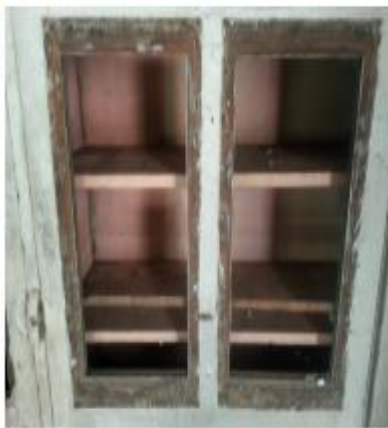
Figure 60: Example of Wythe Punched-Tin and Built-In Pantry from House in Rural Retreat, VA, ca.1830, today only remnants of its tins exist, Photo by Author.
