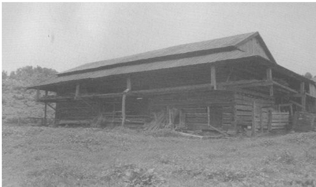
Figure 13: Cantilever Barns on the Western Waters, (Top) Kettering Barn in Rural Retreat ca.1815, (Bottom) Copenhagen Barn on the county border of present-day Wythe and Smyth Counties ca.1830, from John Morgan's "The Cantilever Barn in Southwest Virginia," in Puglisi et al, eds., Diversity and Accommodation , 286-287, with permission of the author.
