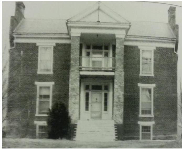
Figure 51: A.C. Moore House, ca. 1825, near the Wythe Lead Mines, Austinville.
