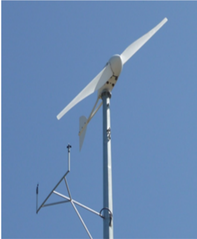
Fig.1 University of Newcastle Australia 5 kW wind turbine, D= 5m
