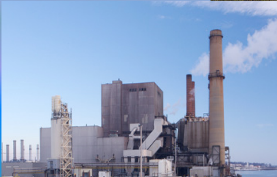
Edge Moor Natural Gas plant, Calpine
