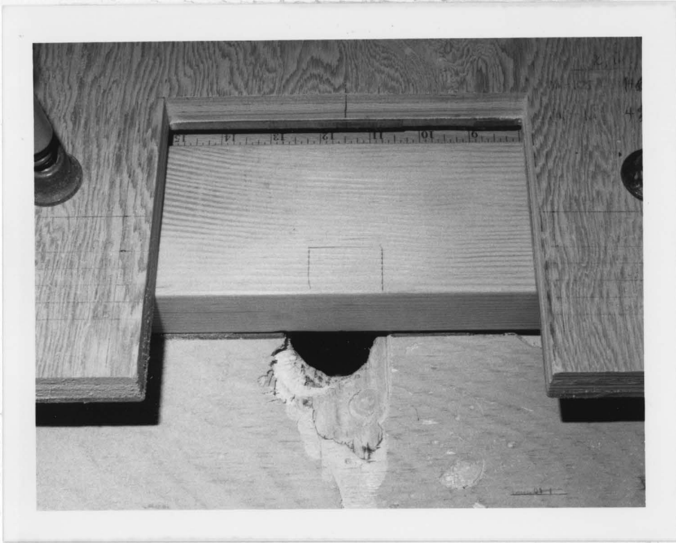
Figure 11. A notching template clamped to a beam to be notched. The notch outline has been sketched on the work-piece.
