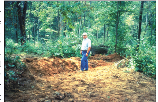
Water bars are large humps that are used to divert water from skid trails.
