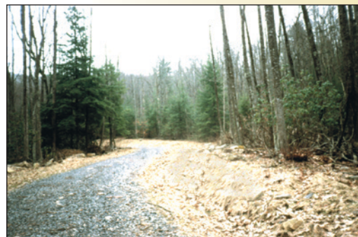
A daylighted road will receive enough sunlight to dry quickly.
