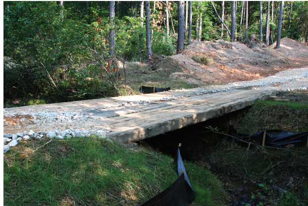
Figure 6: Proper stream crossings are an important part of protecting water quality. Notice that, in addition to the bridge, the stream banks have been seeded to reduce erosion.
