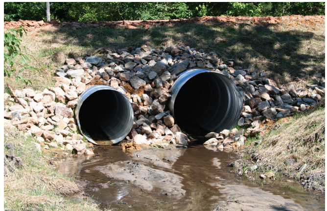
Figure 12: Following Virginia's Best Management Practices helps ensure the protection of water quality. These culverts are part of a well-planned stream crossing.
