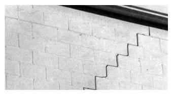
Figure 2. Settlement cracks in a masonry wall that has been subjected to angular distortion due to differential settlement.
