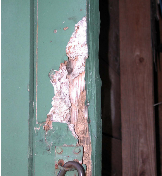
Figure 54. Decay on a door frame
