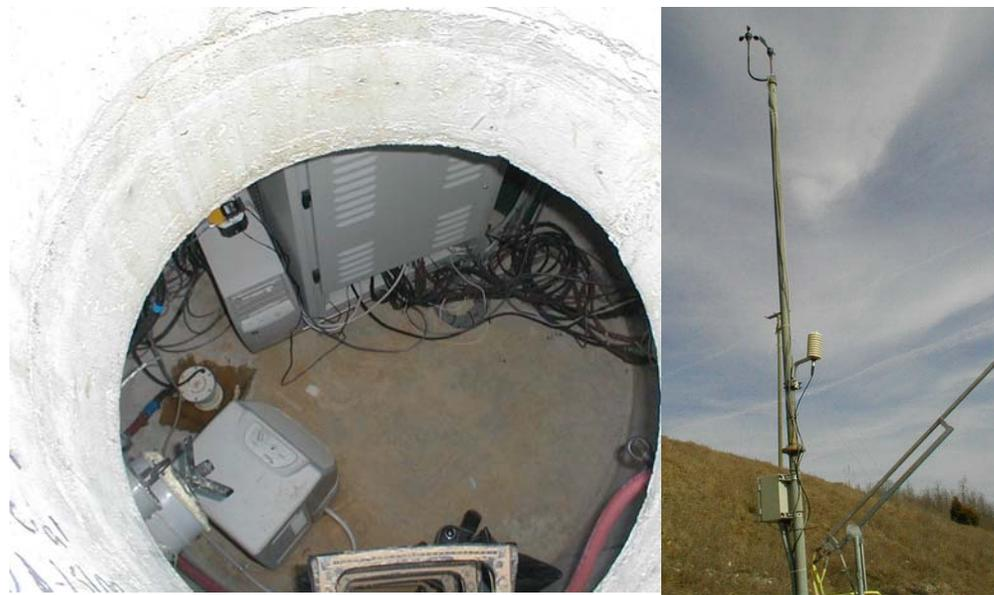
**Figure 58. Bunker with DAS and weather station installed on the Smart Road.**
