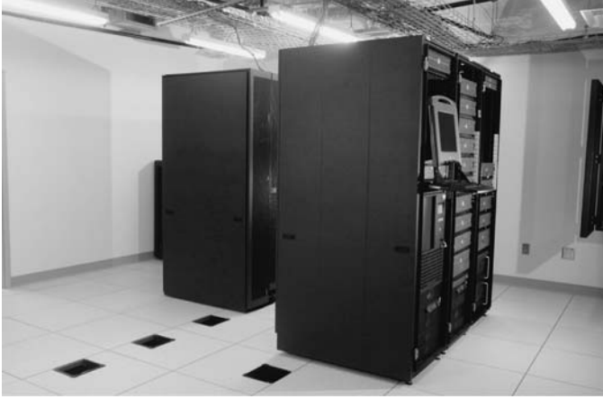
Figure 4.1. Environmentally controlled and secured VTTI data center.
