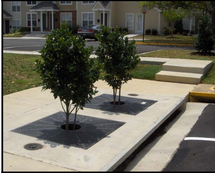
Figure 2. Hollies planted in Filterra® units installed in a parking lot with replicate landscape holly in background.
