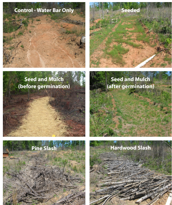
Figure 2. Temporary skid trail closure treatments.
