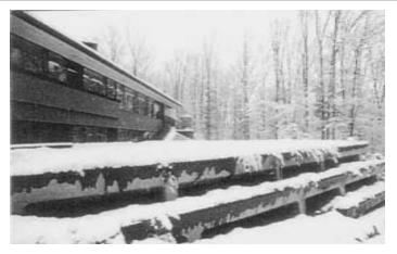
Gottlieb House: The house used pre-fabricated, recycled and ecologically sound materials and was a collaboration between Lois Gottlieb and her son on his house. Above, a pool terrace is supported by a retaining wall of 16-foot pre-fabricated sections used to support highways in Switzerland. Below, a skylight at the ridge of the roof; glulam beams support the entire structure.
