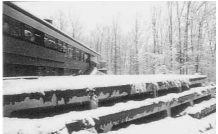
Gottlieb House: The house used pre-fabricated, recycled and ecologically sound materials and was a collaboration between Lois Gottlieb and her son on his house. Above, a pool terrace is supported by a retaining wall of 16-foot pre-fabricated sections used to support highways in Switzerland. Below, a skylight at the ridge of the roof; glulam beams support the entire structure.
