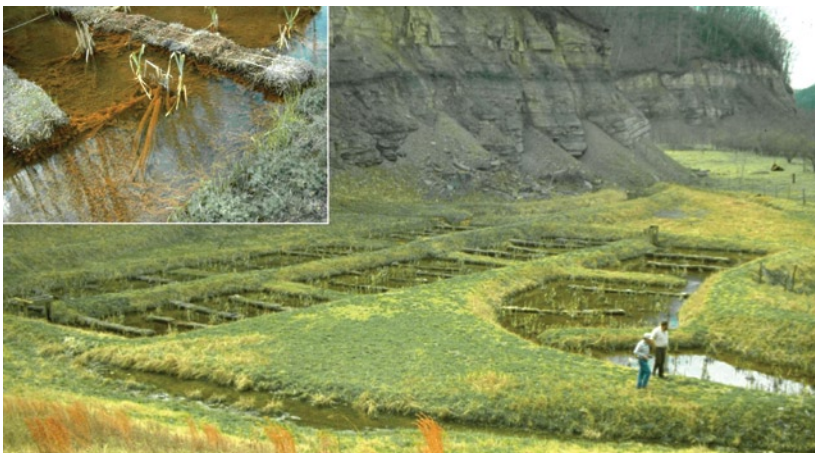
Figure 5. Because poor water quality and low nutrient availability hindered plant growth in this aerobic wetland, haybales were placed to prevent flow channelization and to add biodegradable organic materials that help stimulate alkalinity generation via sulfate reduction. The inset photo shows iron floc accumulating on the biodegradable organic material. Water draining from an abandoned deep mine enters the system to the right of the inset photo, and flows through the system toward an exit at the lower right.
