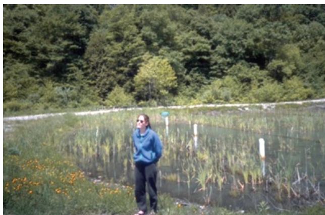
Figure 11. The upper surface of a vertical flow system constructed in 1990 to receive effluent from Westmoreland Coal Company's Pine Branch refuse pile (Duddleston et al. 1992). The vertical plastic piping visible in the background was installed to enable "clean out" of the drainage system, should that prove necessary, prior to the development of the flushing valve concept depicted in Figure 13.
