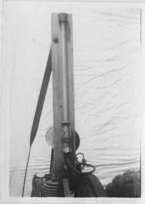
Fig. 6 - Fuel Measuring Device.
