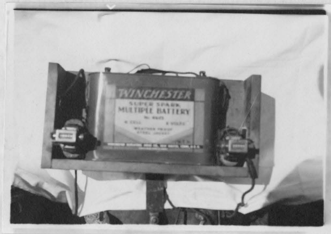
Fig. 5 - Wheel Revolution Counting Device.
