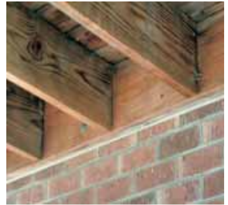
Critical connections along the underside of the deck
