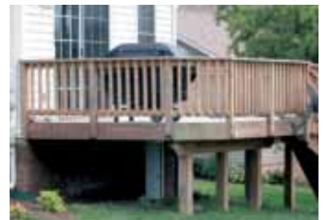
Picket spacing no wider than four inches prevents falling and choking hazards.
