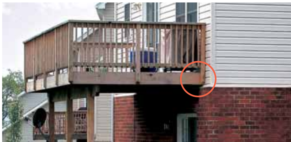
Circled in red is the deck-to-house connection, which is a common point of failure for many decks.
