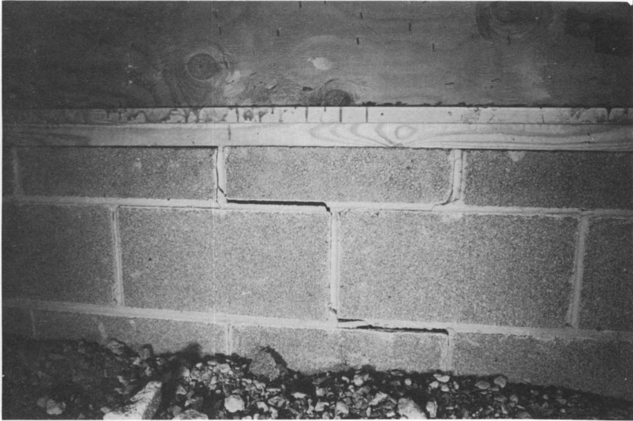
Fig. 10. FOUNDATION FAILURE
