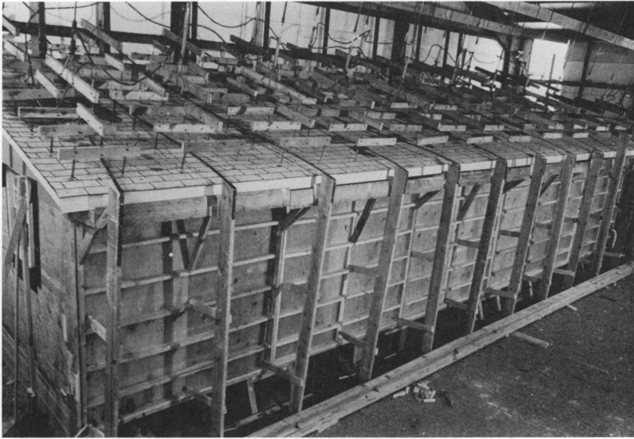
Fig. 5. THE MODULE RIGGED FOR SIMULATING WIND-LOAD TESTING (See Figures 3 and 6).
