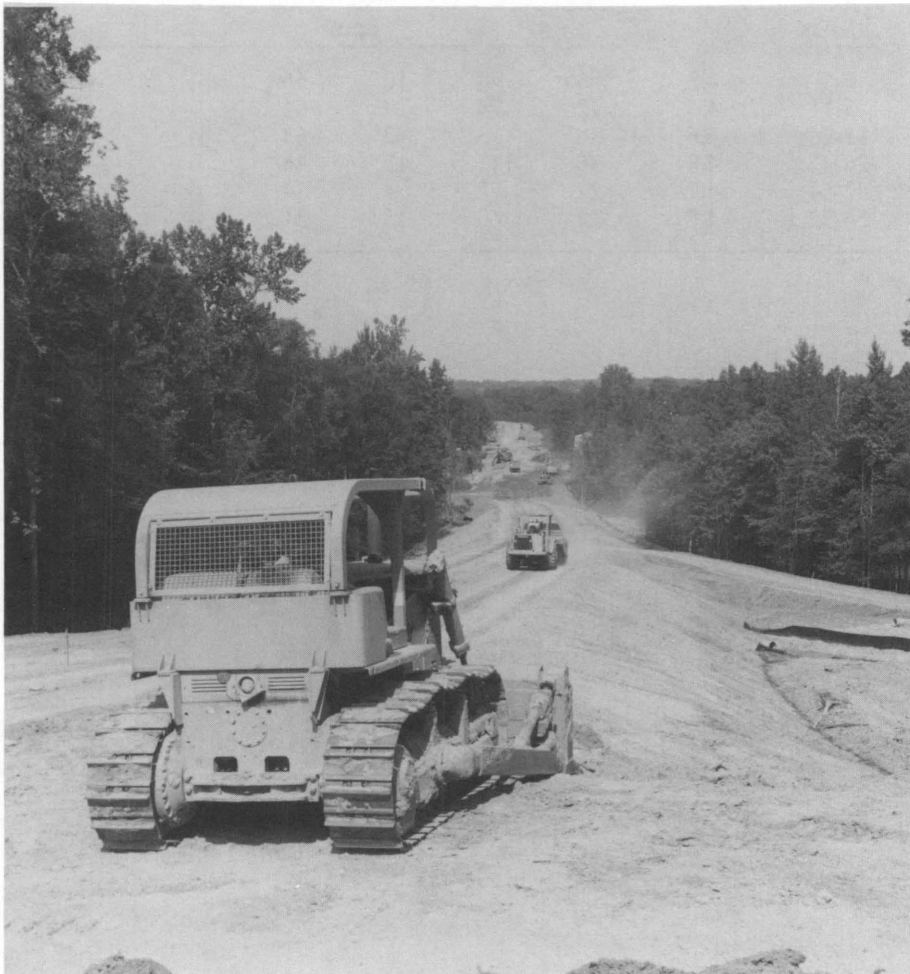
Photo 4. Roadbase materials for VA-106 near Roxbury were borrowed from Nevarc-Remlik gravelly soils.
