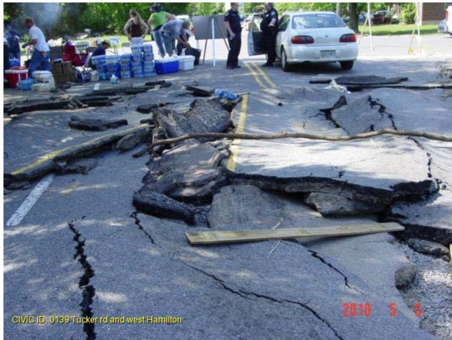
FIGURE 1 Example of Pavement Damage Due to Severe Flooding.
