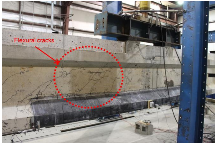
Figure 3.22: Test 3.1 Cracking Near Peak Load
