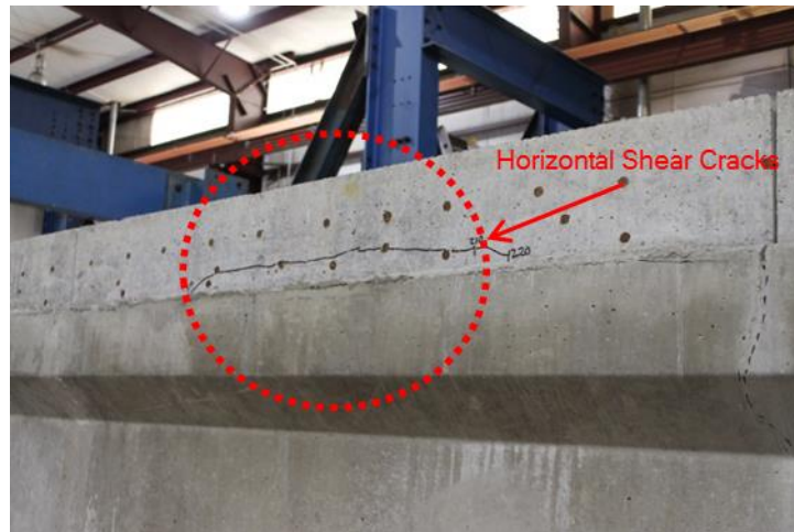
Figure 3.31: Horizontal Shear Cracking in Deck of Test 5
