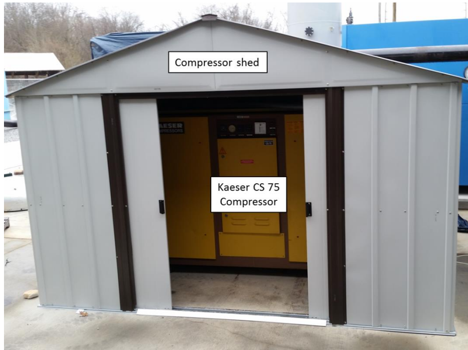
Figure 17. Kaeser CS 75 compressor repurposed to supply shop air at APPL. The shed protects the compressor from rain and snow.
