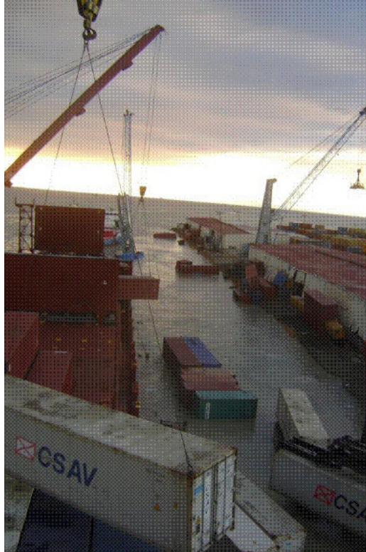
Figure 1.1: Liquefaction during the 2010 M_w 7.0 earthquake caused damage at the Port-au-Prince seaport, hampering relief efforts. (gCaptain 2010) [Fair Use]
