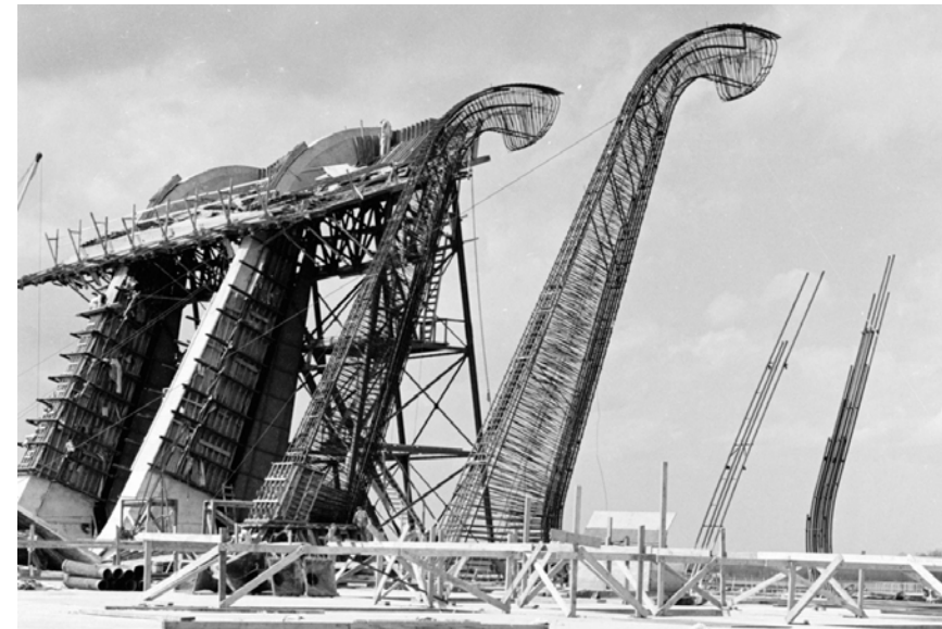
4, Dulles Airport raw structure
