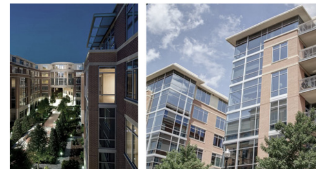
12, Falls Church apartments
