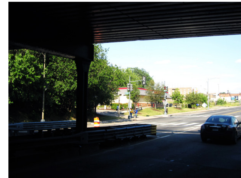
under railroad bridge, Florida Ave
