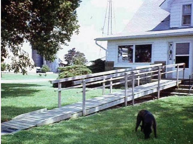
Figure 7. Ramp for improving wheelchair access.
