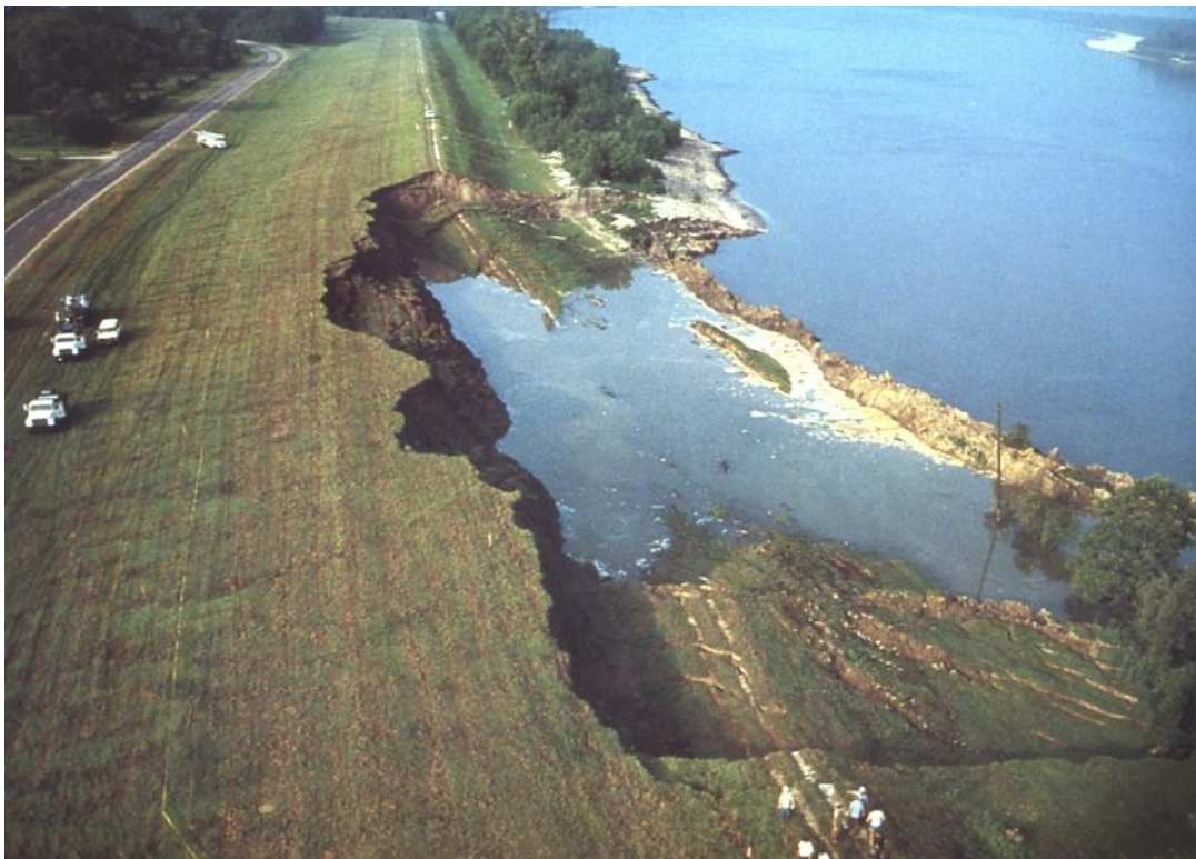
Figure 8-10. Aerial view of Marchand levee failure, looking downstream (from USACE 1984)
