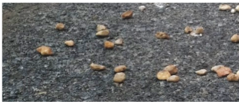
(a) Gravel on road
