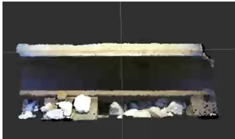
(a) Scan with raised spikes and misplaced ballast
