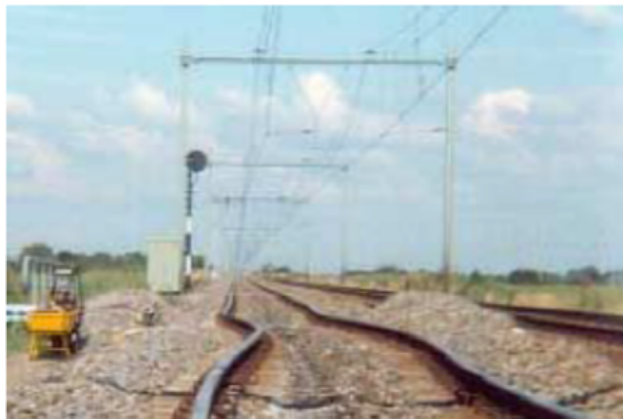
Figure 2.1: Buckling of railway tracks [19]
