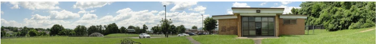
Figure 19: The pathway connection between the Melrose library to the Elementary School in the back of the park. Source: Author
