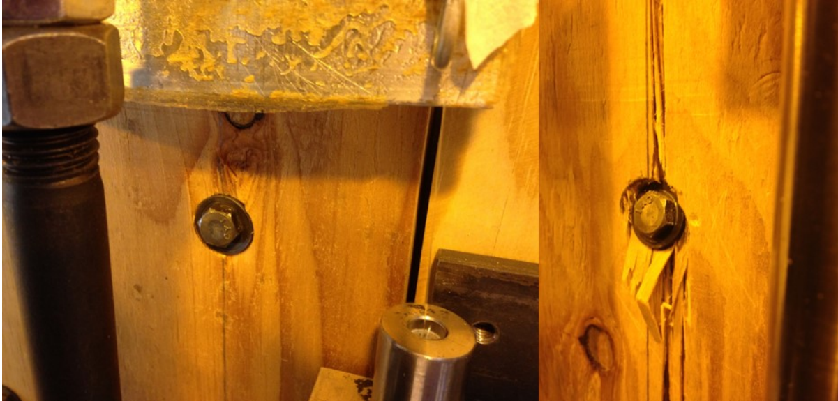
Figure 4-11: Photographs of Fastener Pull Through in the Surface Spline Connection
