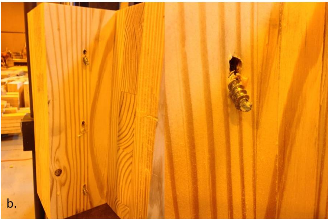
Figure 4-12: Photographs of Observed Failures in Half-Lap Connections
