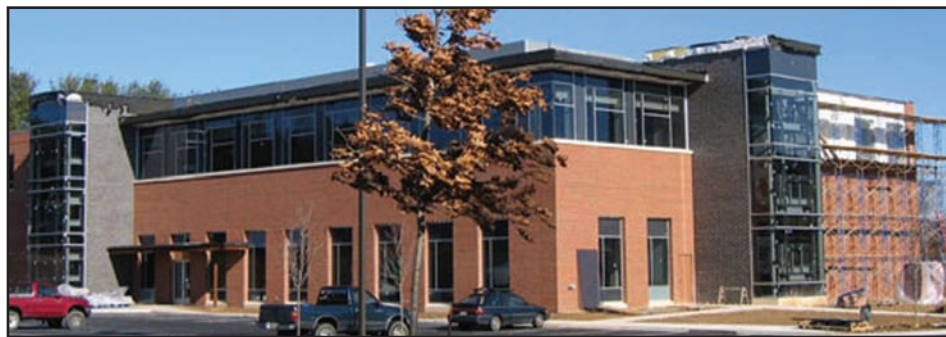
ICTAS A is currently nearing completion within the Virginia Tech Corporate Research Center. This building will house the Nanoscale Characterization and Fabrication Facility (NCFL).
