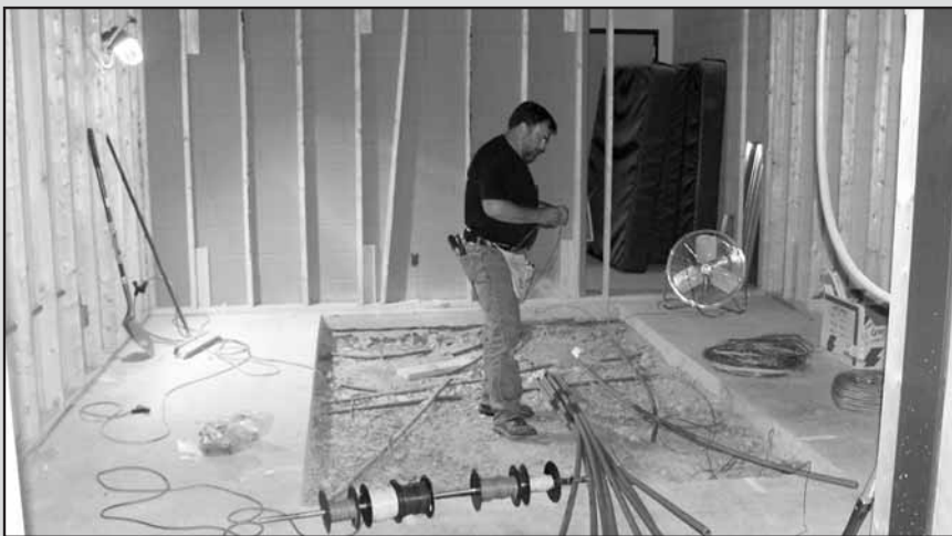
Work is underway on the installation of a standing MRI unit at the EMC. The standing MRI will enable clinicians to accurately image the lower leg without anesthesia. The MRI is expected to be put on line in early 2004. Center officials believe it will be one of the first two such units available in the United States.
