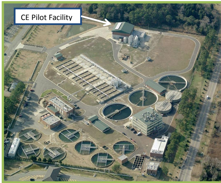
Figure 3 – Aerial Photograph of the Chesapeake Elizabeth Wastewater Treatment Facility. https://www.bing.com/mapspreview . Produced from Bing Imagery, 2015. Used under fair use, 2015.
