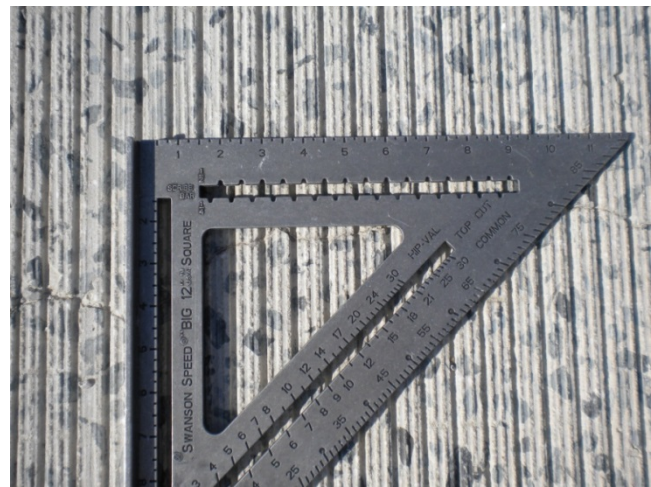
(b) PCC right wheel path, 19 mm ( \frac{3}{4} - inch) groove spacing.
