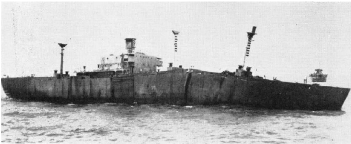
Figure 13 – Failure of Liberty Ship Hull Girder due to Noncontact, Under Keel UNDEX [18]
