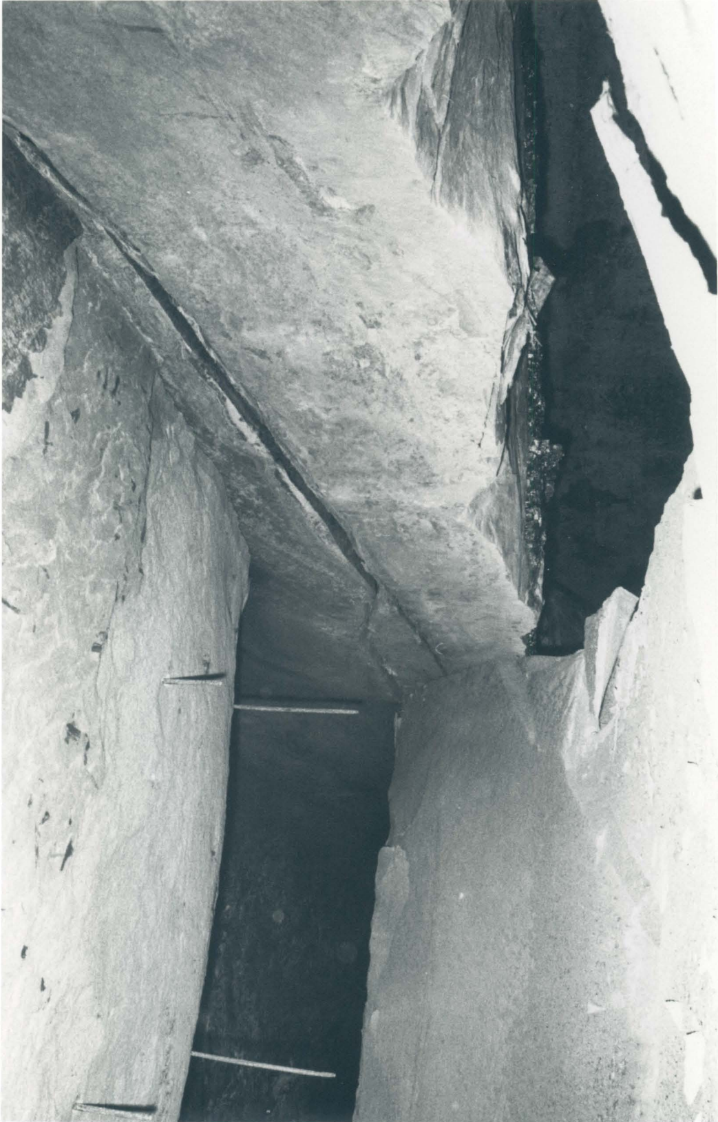
Figure 4.25: Another view of roof fall in Figure 4.24 (photograph by T. M. Gathright, II).
