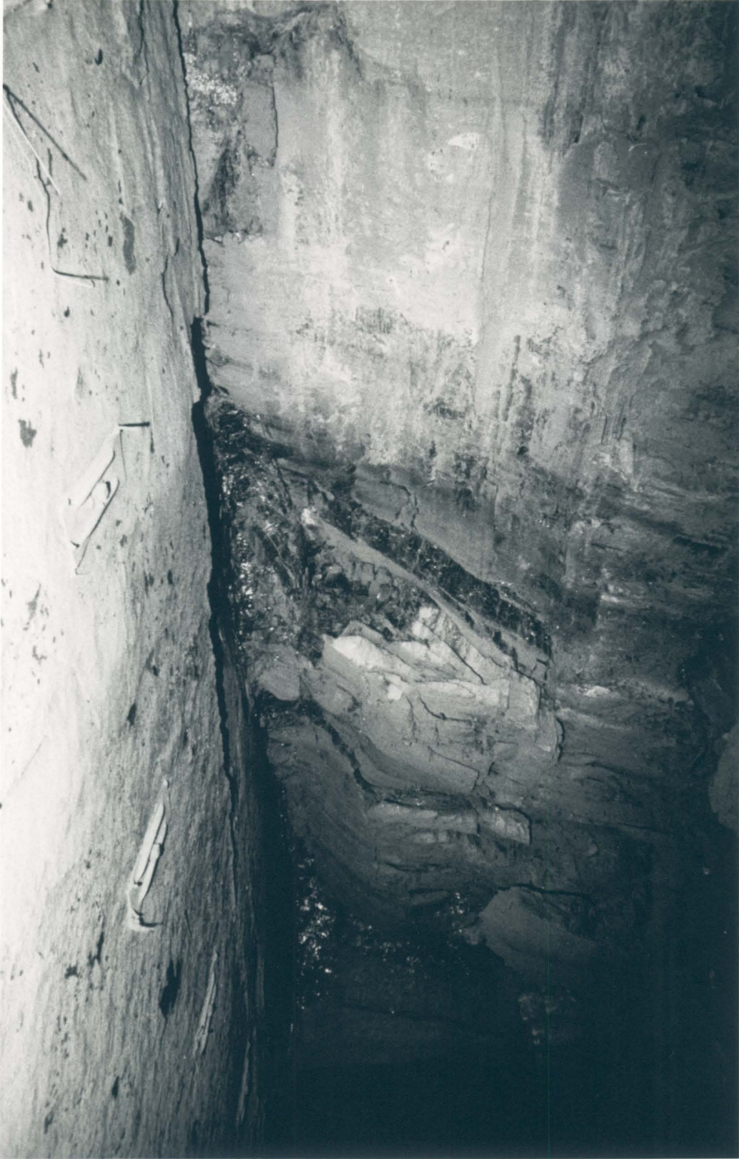
Figure 4.6: Faulted coal beneath massive Sandstone Roof.
