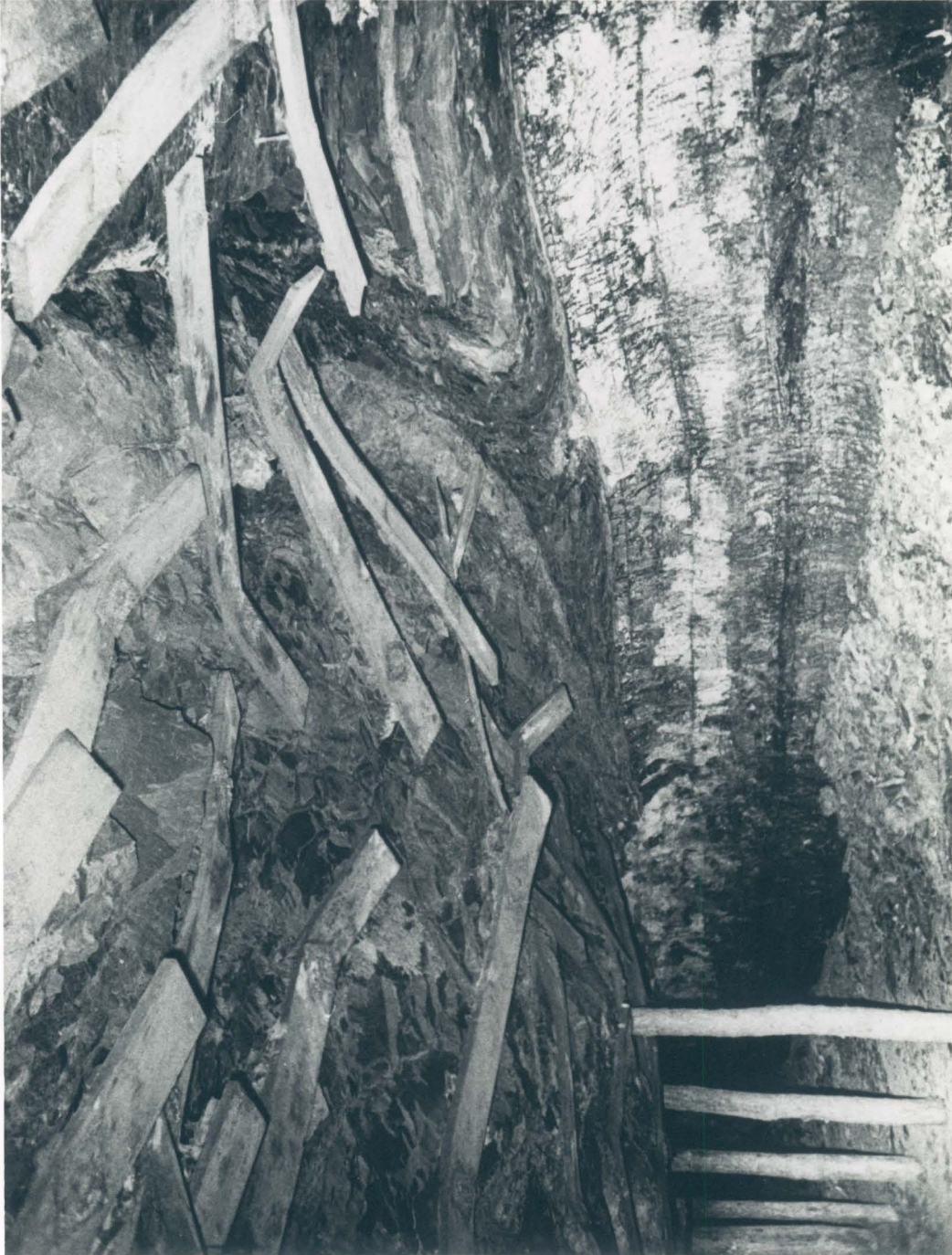
Figure 4.8: Decollement seen in mine roof (photograph by T. M. Gathright, II).
