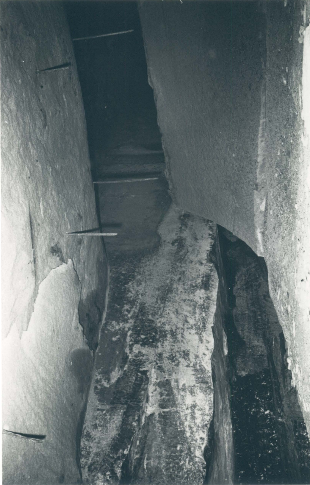
Figure 4.24: Roof fall due to vertical jointing of Sandstone Roof (photograph by T. M. Gathright, II).
